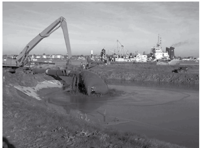
plate 3. Dredged mud being pumped through a pipeline and into a retaining bund to settle out.
