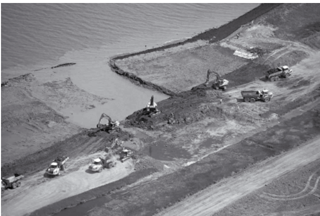
plate 2. Final breaching work (8000m 3 of material removed during a seven hour tidal window).
